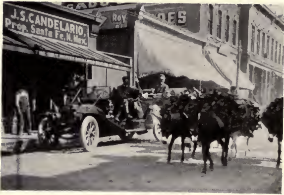
"Compra Llena," buy wood, is the cry heard, like the call of the "old clothes" man of Eastern cities, in Santa Fe, New Mexico, as the Indians drive their laden burros through the streets
